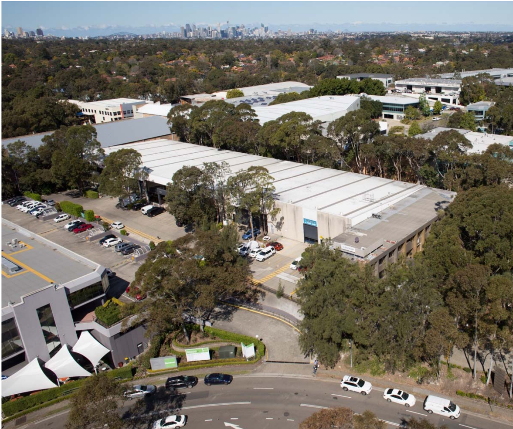
Aerial view of 7-9 Orion Rd, Lane Cove
