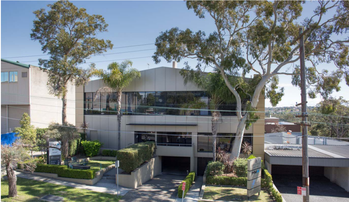
Image: 13 Sirius Rd, Lane Cove NSW
