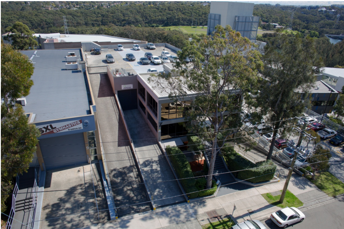
Image: 7 Sirius Rd, Lane Cove NSW
